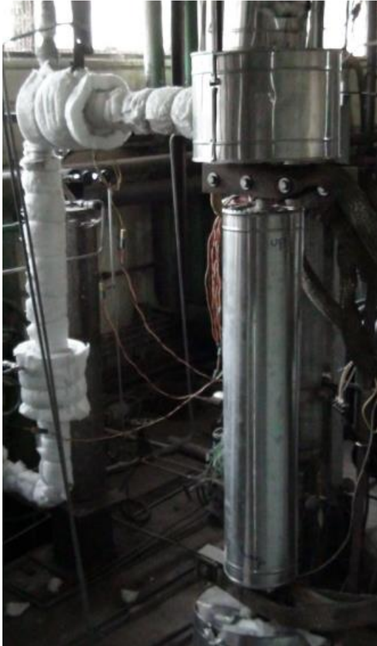
Figure 54 The High Pressure (100 bar, 300 C) CHF film flow rate facility
