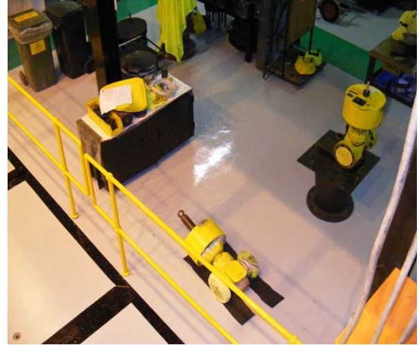
Photograph 3e – Properly designed lay down areas for storage with good access.
