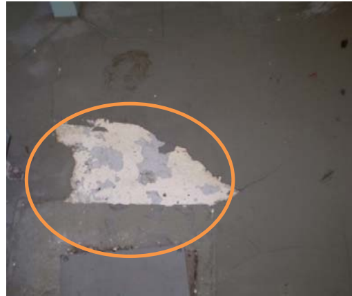
Photograph 2b - Poor building standards leading to foreign material generation.
