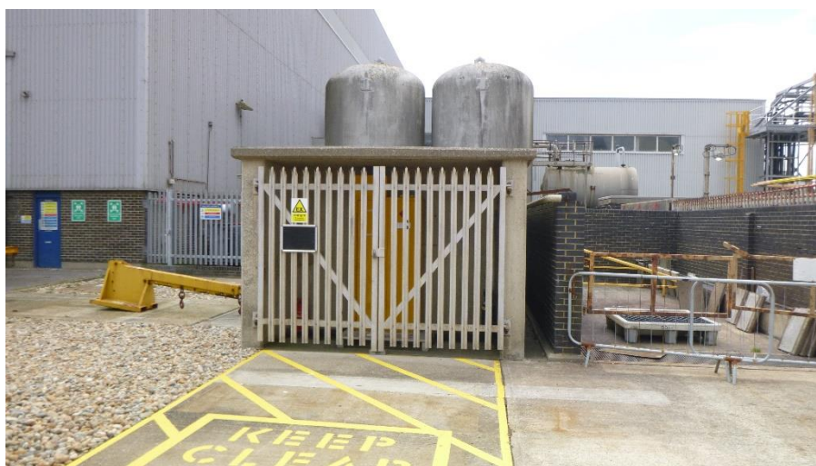
Plate 3: Hard standing and industrial buildings within Area A of the Works Area
