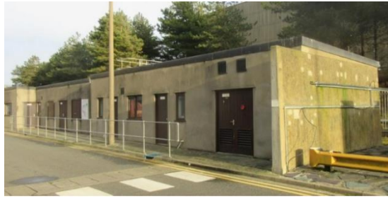
Photograph 5 - Breathing Apparatus (BA) Set & Training Facility
