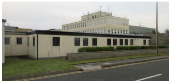
Photograph 7 - Administration Building Extension
