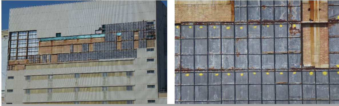
Reactor 2 south face following phase 1 repairs to make the buildings safe
