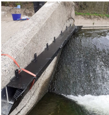
Eel Pass over Milnby Weir
