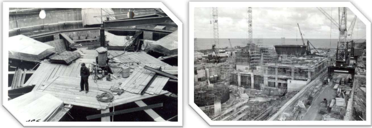
Photographs 30 & 31 – Wylfa site during construction circa 1965
