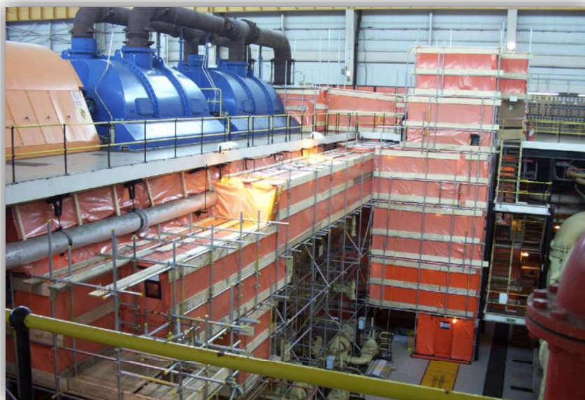
Photograph 3 - Turbine Hall Asbestos removal at Hinkley Point A Site
