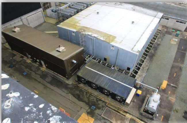
Photographs 10 & 11 Back up feed system, tertiary feed pump house/water tank/fuel tank, EOS double bank radiators/fuel tank before and after
