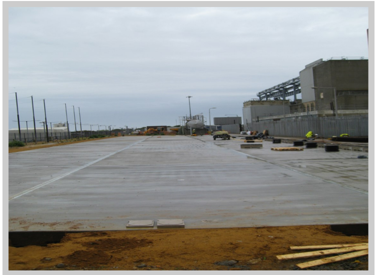
Figure 9: New Waste Slab Storage Area nearing completion.
