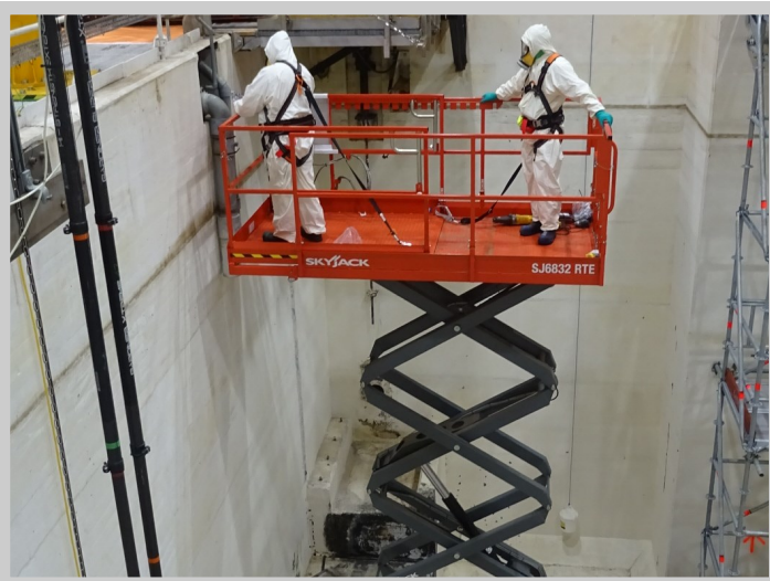
Figure 8: Deplanting activities being carried out within the Cooling Ponds.
