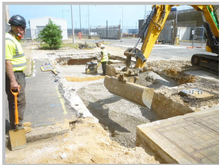
Figure 4: Sub-surface Voids Repair Works
