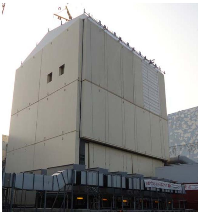
**Figure 1 : Containment structure enclosing reactor 1**
