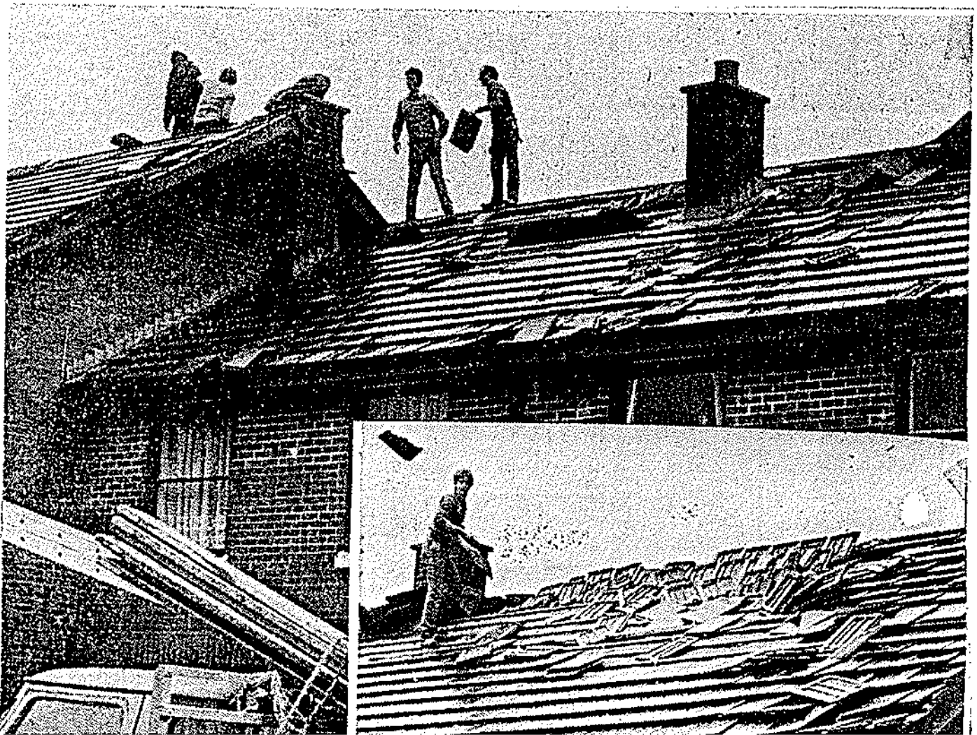
Figure 7. The verge tiles removed from the gable ends of these houses together with more general damage to the roof of the middle house suggests T1 winds (25 January 1971, Welling, Greater London). Figure 8. Roof damage in Belfast, 26 September 1982, indicative of force T2 wind-speeds.
