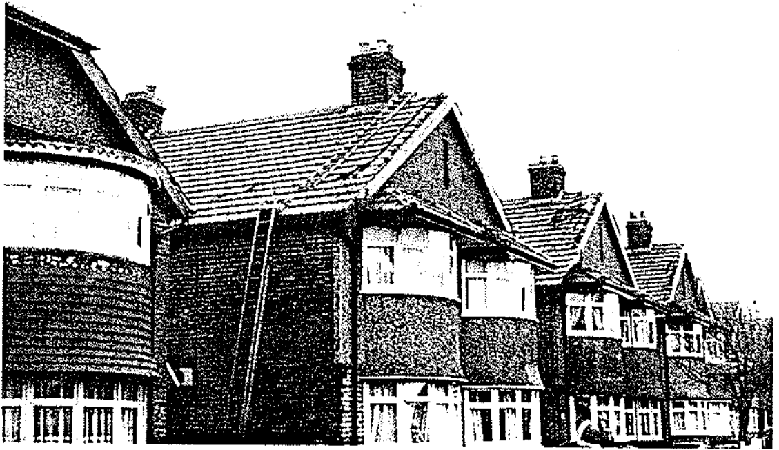
Figure 7. The verge tiles removed from the gable ends of these houses together with more general damage to the roof of the middle house suggests T1 winds (25 January 1971, Welling, Greater London). Figure 8. Roof damage in Belfast, 26 September 1982, indicative of force T2 wind-speeds.
