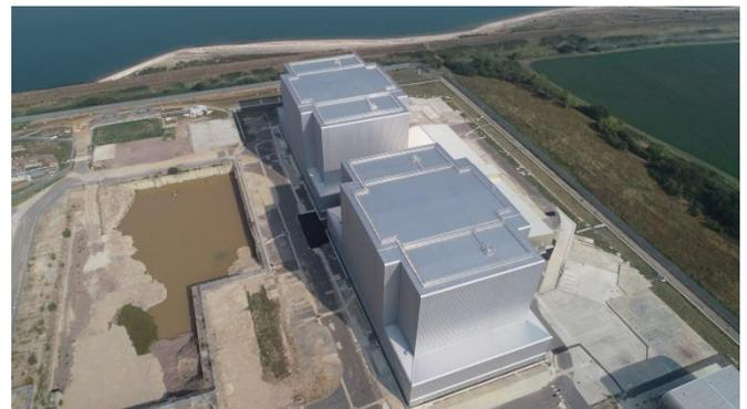
**Figure 5: Image of the Reactor Safestore Weather Envelopes**
