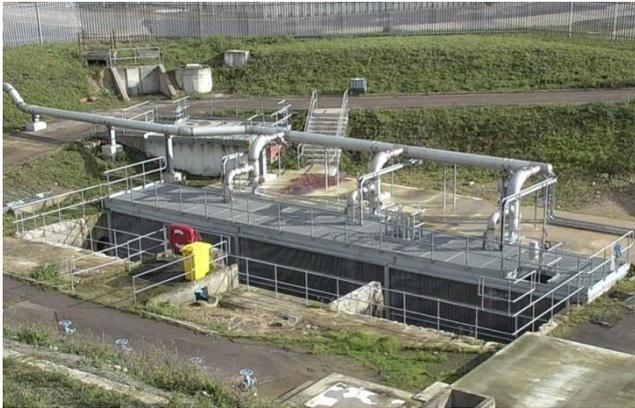
**Figure 7: The four pipelines inside the Main Drains Pit**
