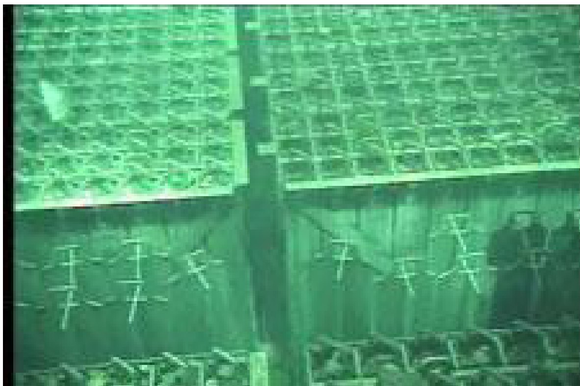
Figure 9: Condition of the Spent Fuel Pool (Reactor Unit 4)
