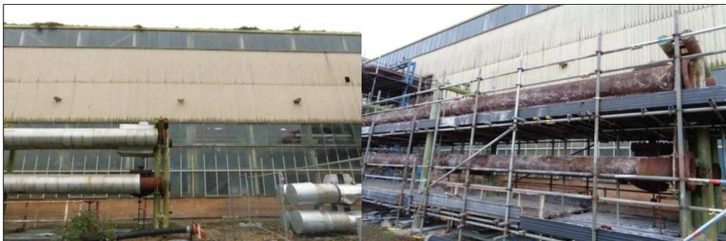
Fig 1: Steam pipes, before and after removal of asbestos insulation.
